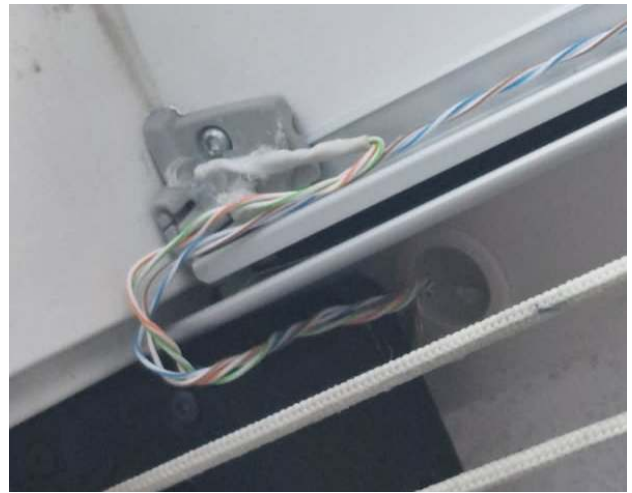
Figure 14: Reed sensor mounted on window frame in lower position, with other cable leading to upper sensor
